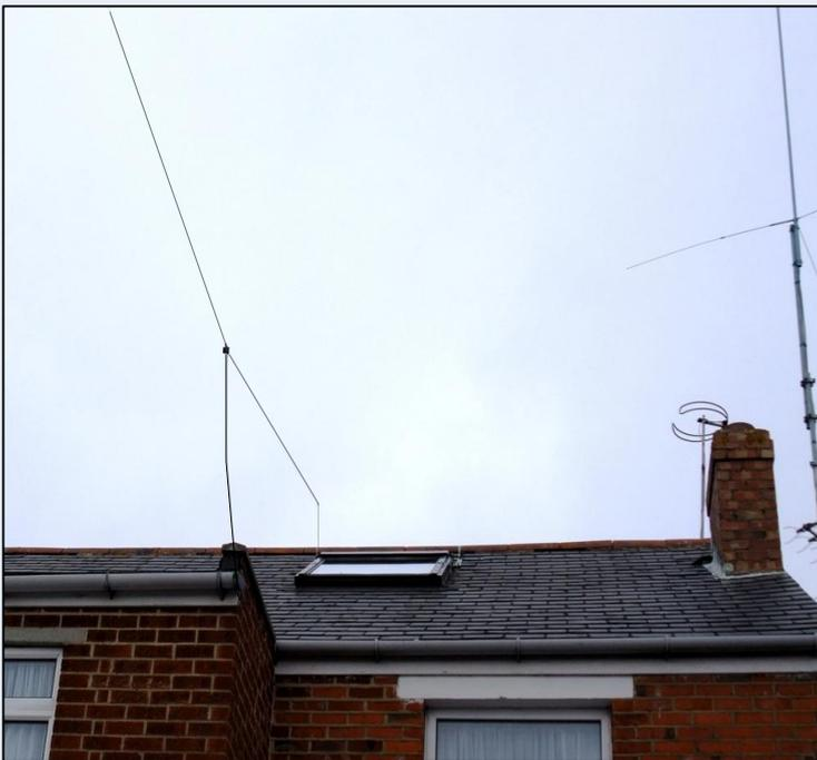
The K1POO antenna has the great advantage for me that the coax feed is very near the house, so it can hang down almost directly outside my window. My garden is only 16m long, so the antenna's shorter end is over the house's roof at 9.5m AGL and the longer end slopes down the garden to a washing line post and fiberglass pole with a combined height of 8.5m. The last 1.5m is bent down at 60 degrees at the end.
